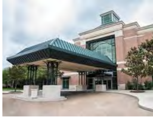
Northshore Rehabilitation Hospital
